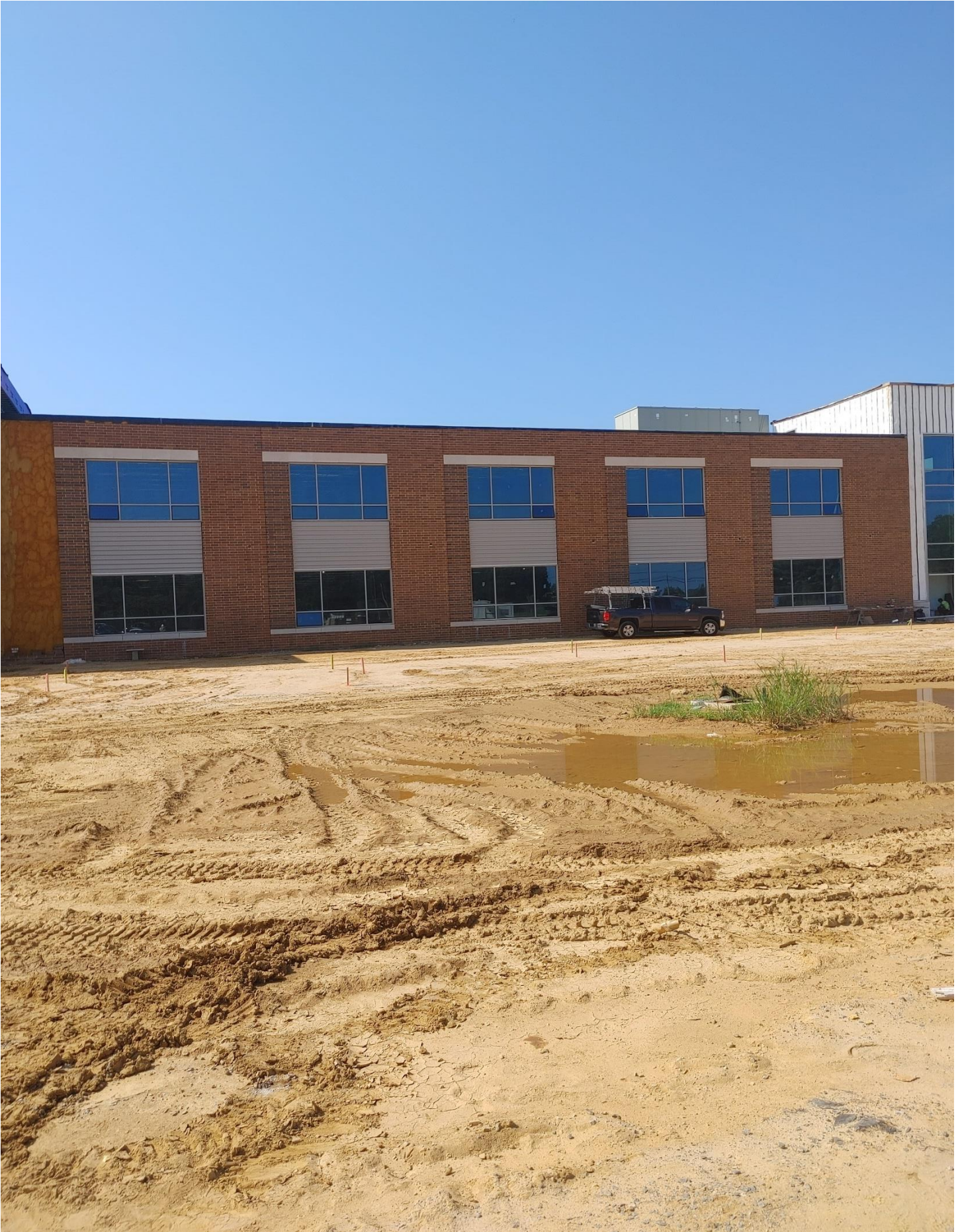
Photo 1 - Metal Panels install on the North side of Area B.
